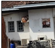
Image: physical aspect of the building – the wall of the post office
