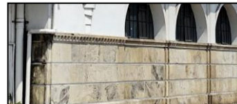
Image: physical aspects of the foundation building of the BAT Building
