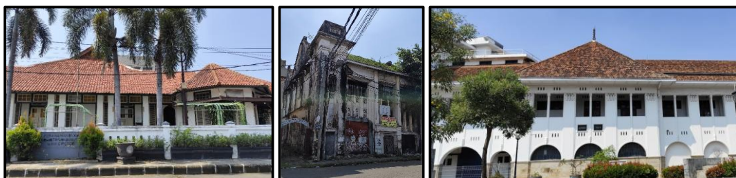
Image: The location of the Cultural Heritage building where inundation often occurs
