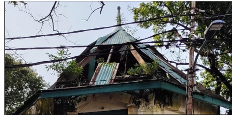
Image: Physical aspects of the building – roof Gedung bunder kebumen Building, Kebumen
