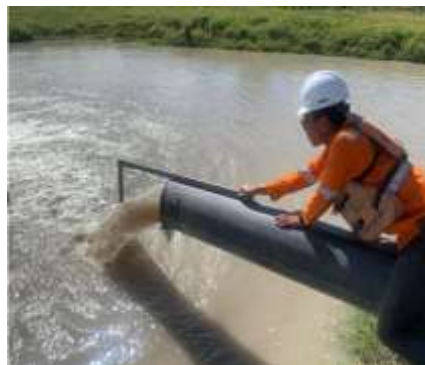
Figure 2. Existing Conditions of Manual Discharge Data Retrieval Using the Flowbar
