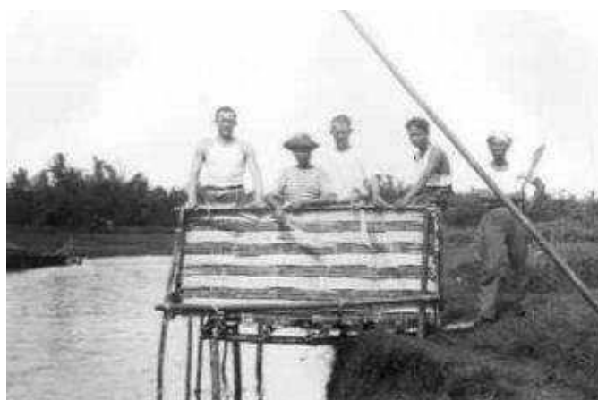
Figure 4. Latrine construction in Kali Mas Surabaya
