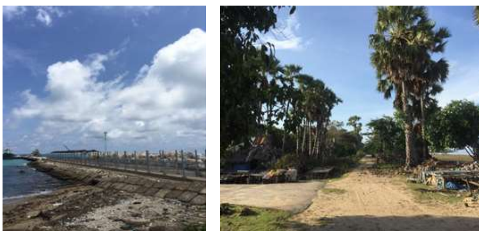
Figure 5. Access to Oseli Village
